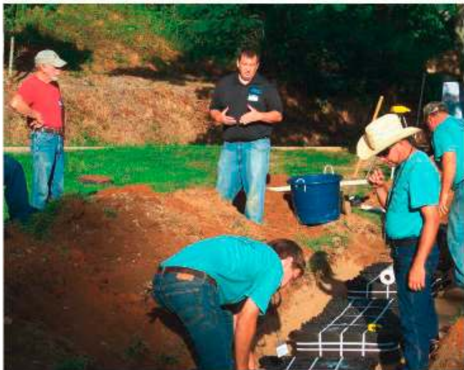
ABOVE: Gravelator Systems owner Harold Kilgore (right) and senior field technician Heath Kilgore apply the second coat of tar and polyethylene film to the dose tank to waterproof it. RIGHT: A crew installs primary treatment modules with orifice sleeves atop them. Eljen representative Jim King explains the procedure to other contractors.
