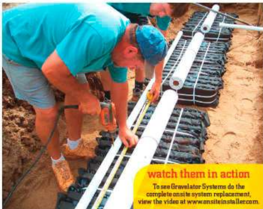
Harold Kilgore (left) and Justin Kilgore drill 0.25-inch orifices in 1.5-inch PVC low-pressure pipe.
