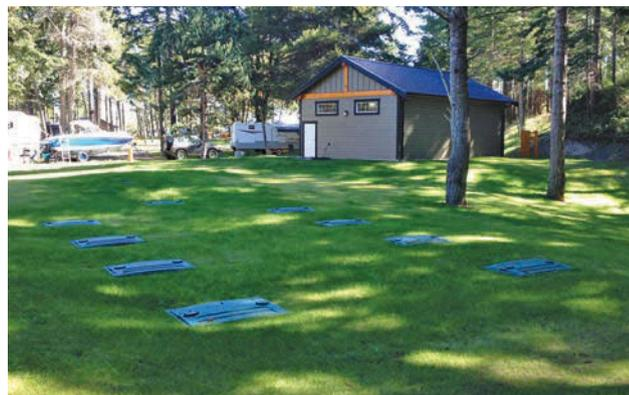
filtering media. The modular design offered the required low footprint, as well as all maintenance, discharge and budgetary requirements. The system provides a permanent and durable solution that treats wastewater without requiring relocation or excavation. At the end of its useful life (up to 15 years), the used filtering media is removed and replaced via the cover and its 10-year warranty is automatically renewed.
