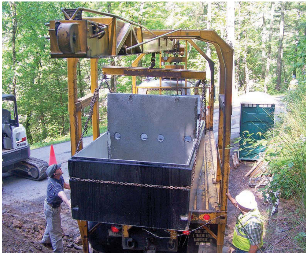
BELOW: Ray Matchen, president of Nix Septic Tank Co., and Harold Kilgore unload the custom 1,500-gallon lowboy combination septic tank.
