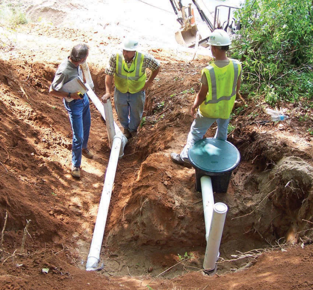
ABOVE: Steve James (left), Rabun County Environmental Health Department manager and onsite inspector, confers with installer Harold Kilgore (center) on the job site. Kilgore worked closely with James during the process.
