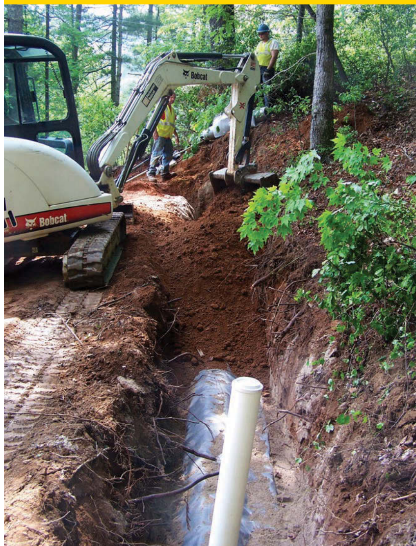
BELOW: Building a road alongside the bottom trench enabled Harold Kilgore to evenly distribute sand and topsoil, minimizing the amount of manual labor to level them.
